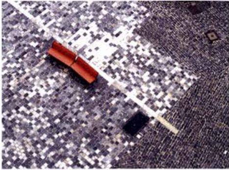
Stone Pavers at Water Feature
